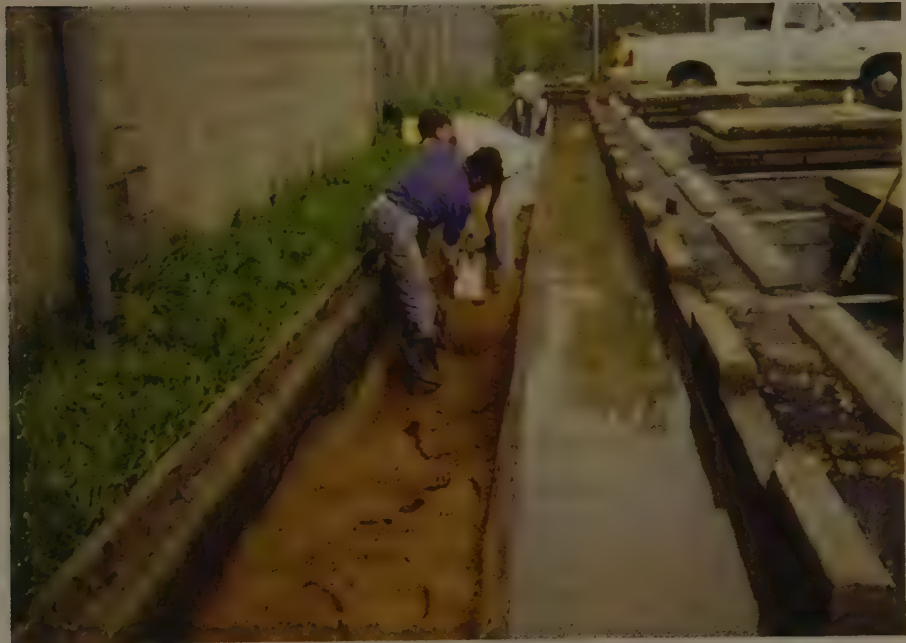
Figure 14.12 Sand Filter Installation at the Perimeter of Parking Lot. Note pretreatment trough and curb-cuts for drainage from lot. Source: Commonwealth of Virginia (1999).
