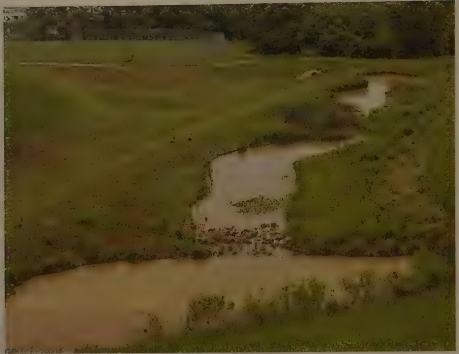
Figure 14.9 New Stormwater Wetland with First Signs of Wetland Vegetation. Source: Commonwealth of Virginia (1999).
