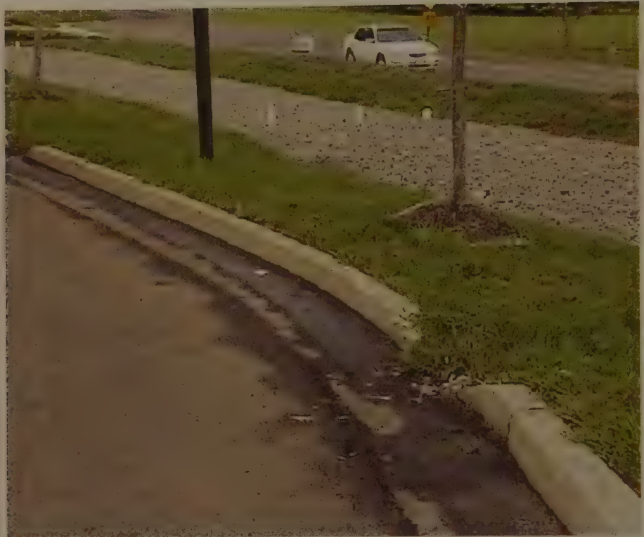
Figure 14.14 Newly Installed Parking Lot Infiltration Trench. Source: Commonwealth of Virginia (1999).
