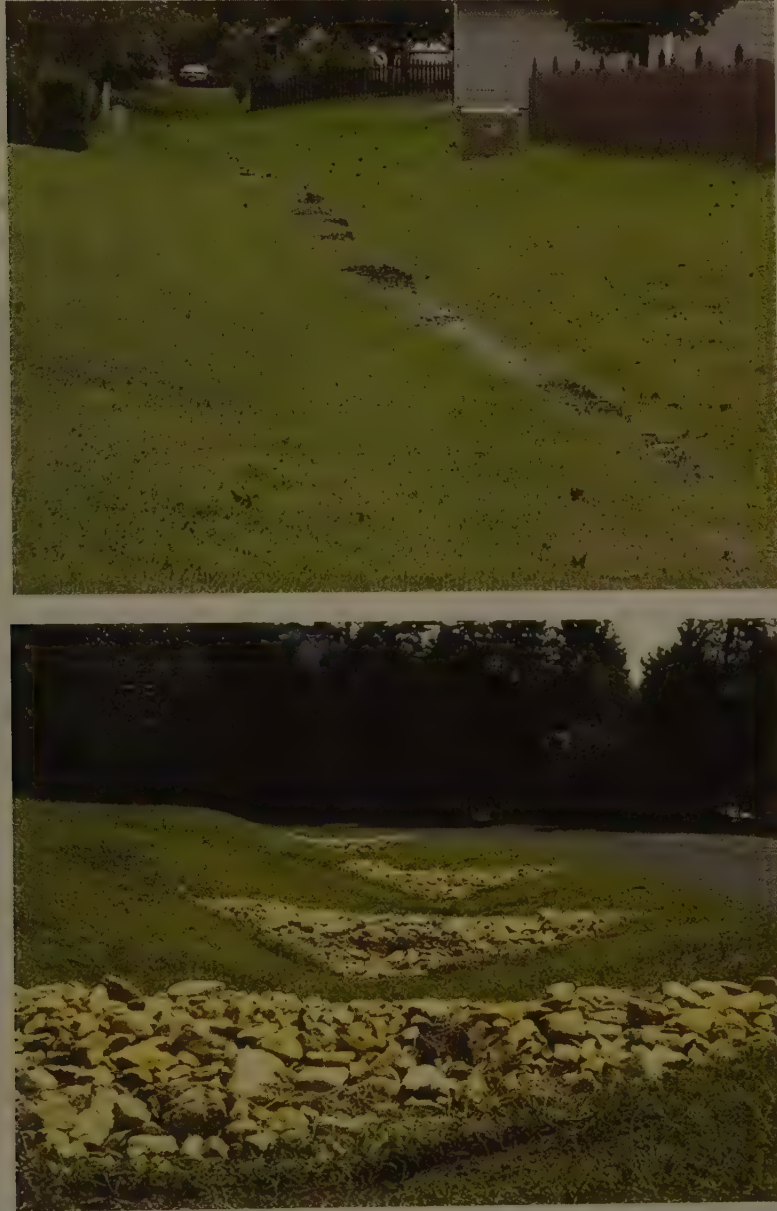
Figure 14.15 Open Channel Swale and Check Dams. Source: Commonwealth of Virginia (1999).
