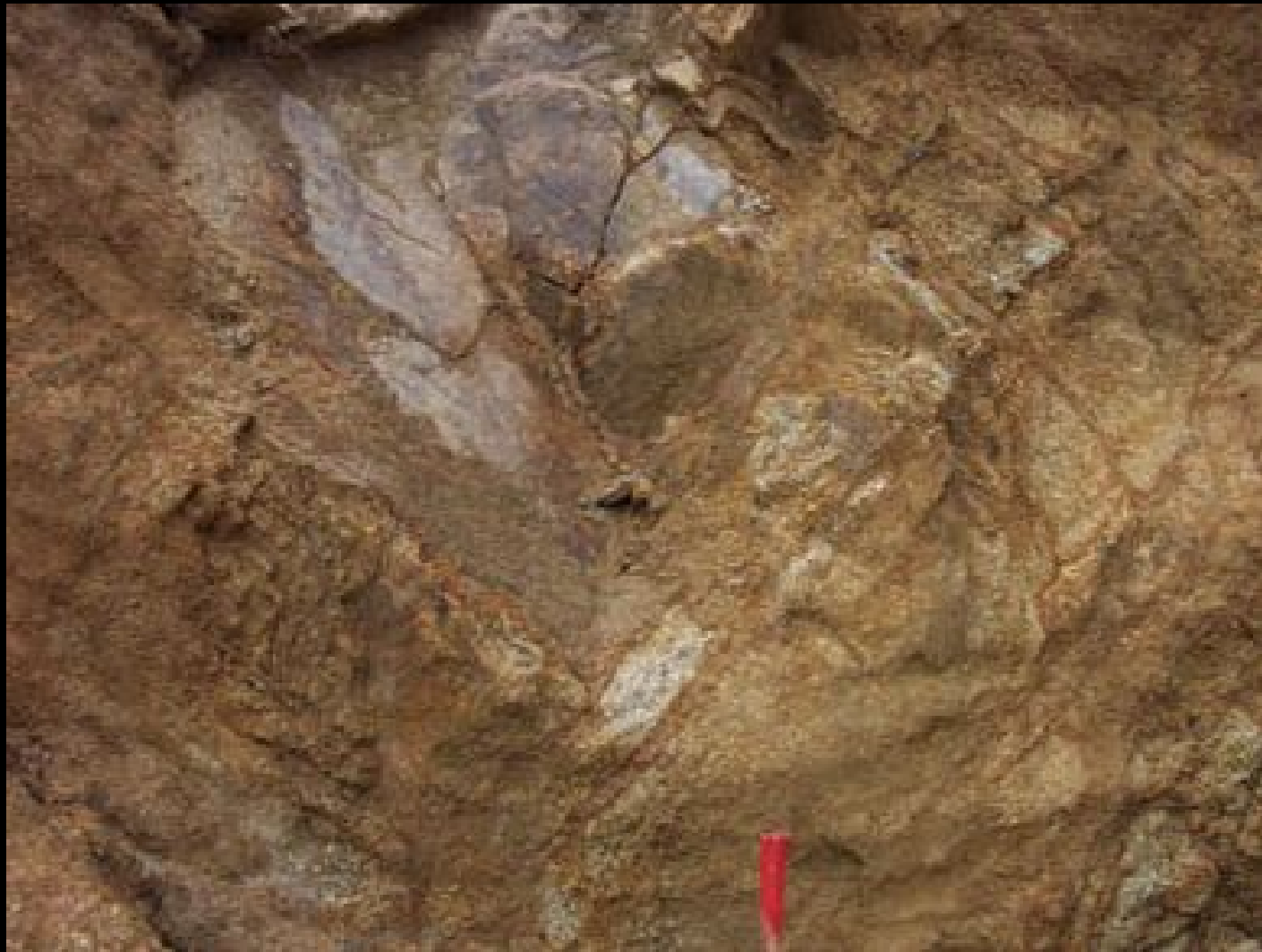
Weathered rock (Gred V)
