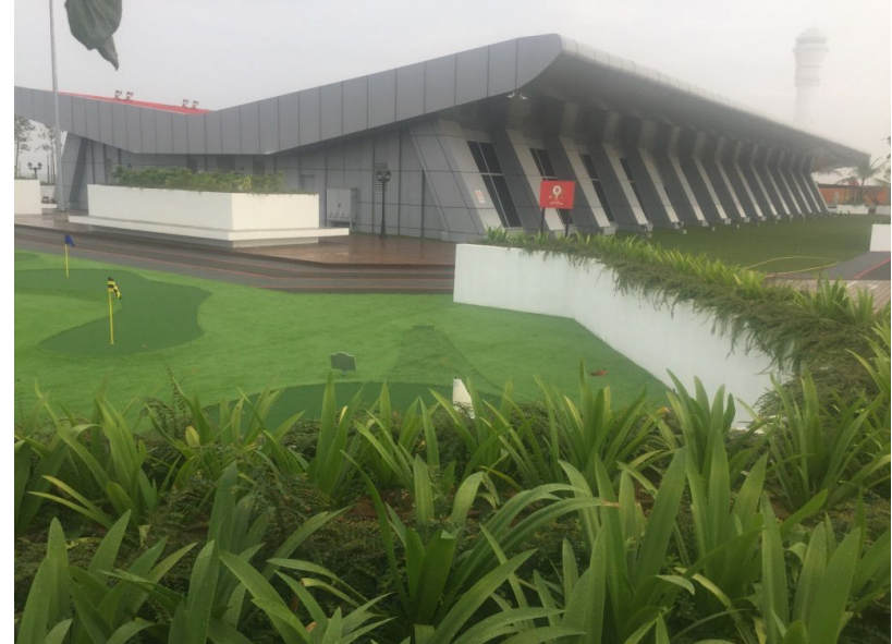
Recreational area (Roof top )
