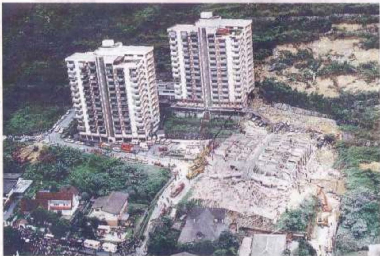
TERRIBLE DISASTER: The two collapsed blocks of the Highland Towers condominium is shown in this file photograph taken on Dec 11, 1993.
