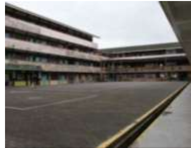
Courtyard (paved area)
