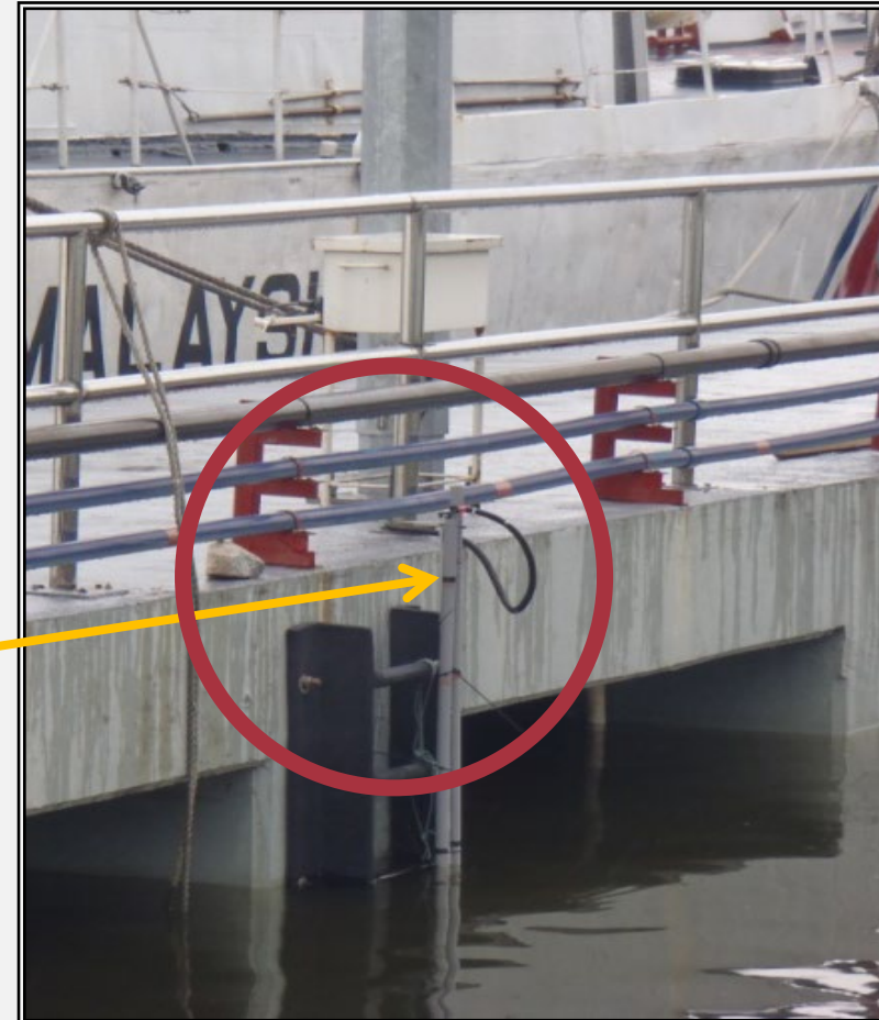
Tide Gauge Installation
