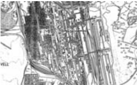
The legacy of the Ravenscraig steelworks (shown here in 1922) is a site largely constrained by sub-surface structures
