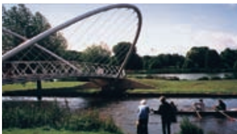
Ouse Bridge, Bedford (Architect: Chris Wilkinson)
