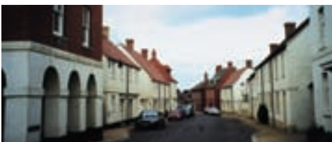
Traffic calming is designed in from the outset
