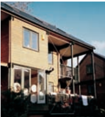
Walter Segal – designed self-build social housing in Lewisham, London
