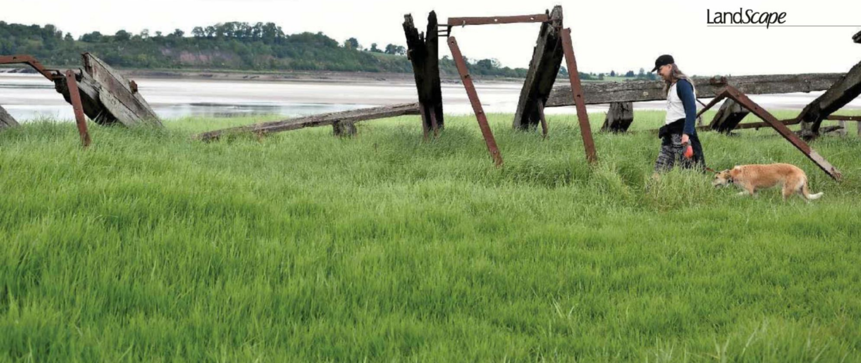
The bare bones of the once imposing triple-mast schooner, the King. Made of both wood and iron, today she is one of a very few survivors of boats made of a composite construction method, used for only 40 years.
