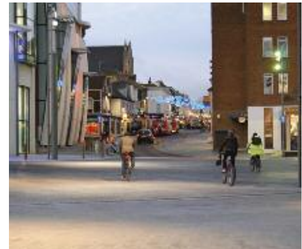
Design detail: Raised bus borders are 165mm high in order to cope with bus access. Bus clearways, if required, are delineated with vanilla blocks instead of yellow lines: where possible material, textures and colour are used to give visual and tactile clues to footways and carriageways. Glass beads in the kerbs glow like cats' eyes at night. In future, double and triple kerbs, along with more sophisticated transitions between footways and kerbs, could be used to create interim spaces for cyclists, pedestrians and the visually impaired. There are many design implications around creating more accessible environments that designers are only beginning to be aware of, hence the need for ongoing workshops, and study exercises
