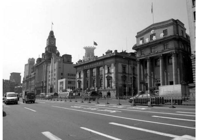
1.3 Deteriorating public space: The Bund, Shanghai
