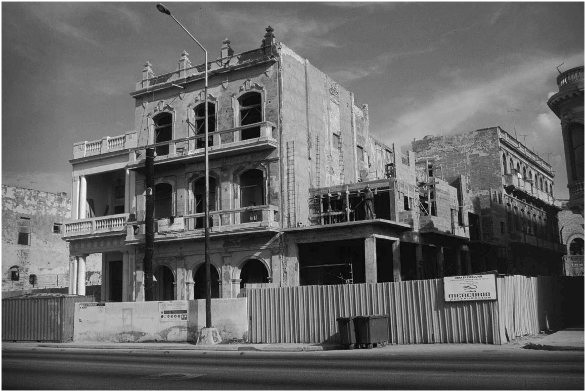
9.4 Ongoing restoration project, Havana.
