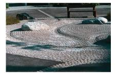
Paved basins show how the rainwater drains away.
