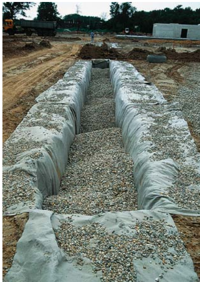
Constructing a swale system between parking spaces
