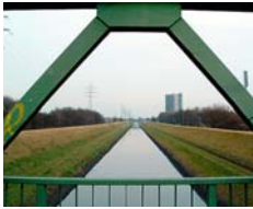
The Emscher today – simply an open sewage channel
