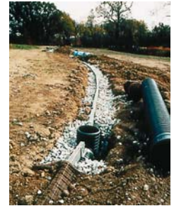
Soakaway trenches for rainwater
