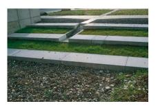
Rainwater is stored temporarily in the sloping avenue open spaces and then runs down to the bottom of the slope in a little stream.
