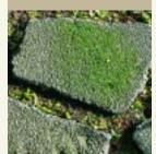
Broken concrete from demolition projects is commonly available yearround, usually free if you can haul it yourself, or delivered for a fee. Broken concrete can be laid similar to stone or other pavers, to create a flagstone-like path.
