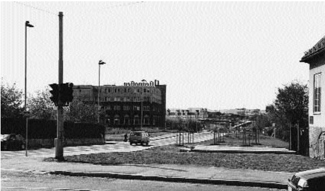
Figure 5.58 Gamle Oslo: conversion of major road into a linear park.
