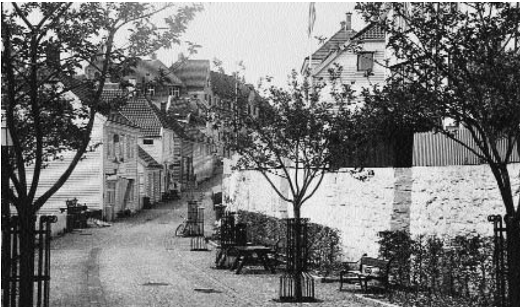
Figure 5.66 Old Bergen, traffic calming.
