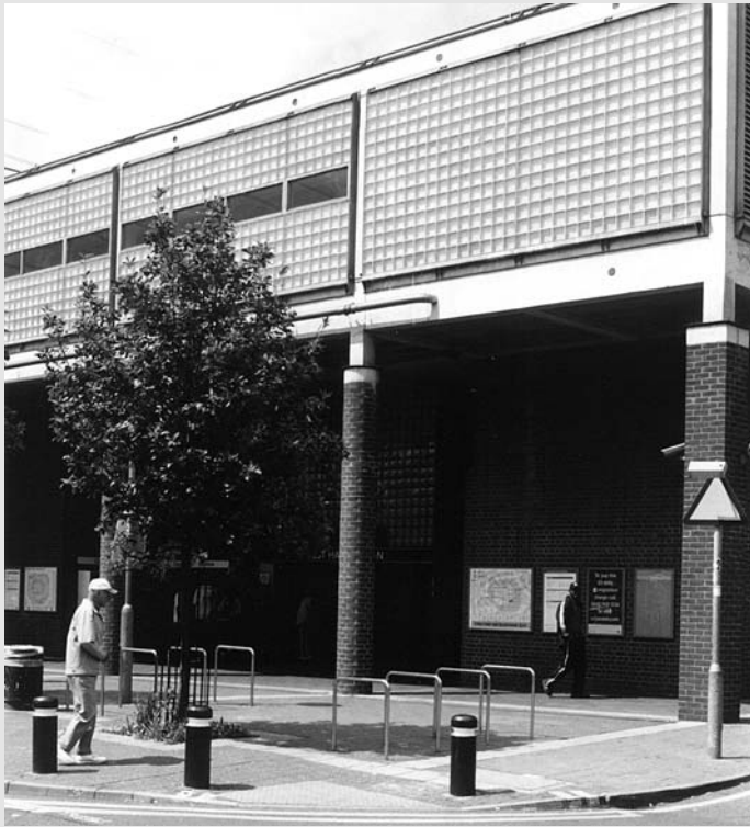
Figure 10.17 The Square at West Ham station.
