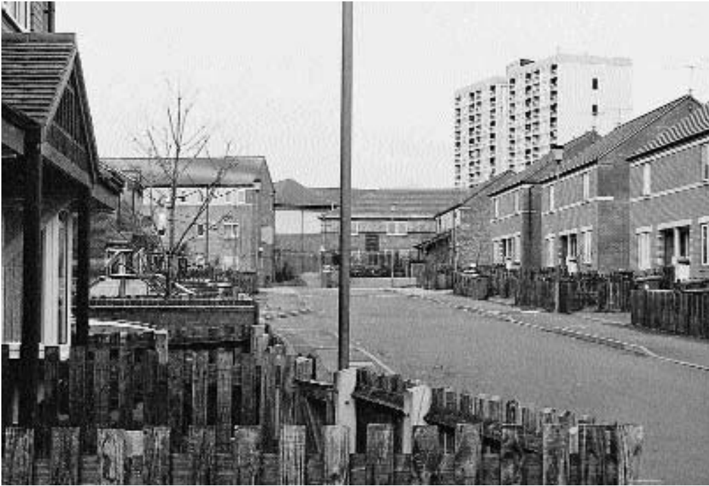
Figure 3.2 Radford. A return to a street architecture after demolition of 1960s deck access flats.
