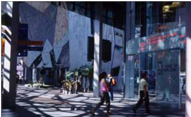
Buildings and venues such as the refurbished GPO (top) and BMW Edge at Federation Square (above) offer new experiences, respectively, in shopping and public events.
