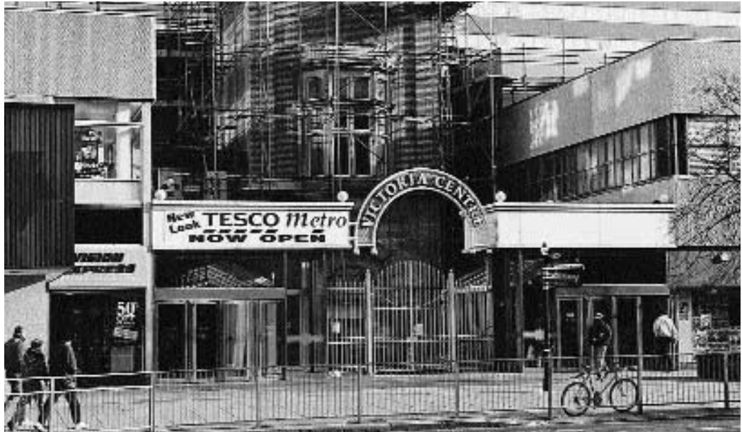
Figure 3.15 Entrance to The Victoria Shopping Centre, Nottingham.
