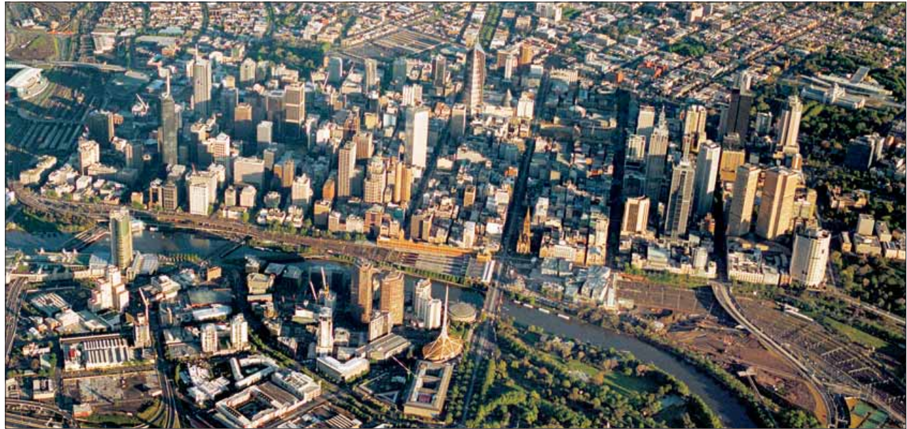
The 40 metre height limit over the retail core area is clearly apparent in the city's physical form, centred on Swanston Street.
