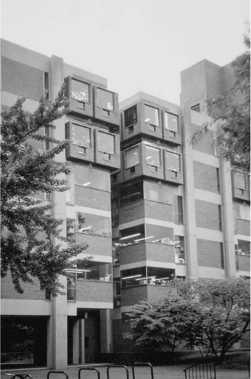
3.8 The laboratory at Penn State University by Louis Kahn. This is a sophisticated piece of architectural manipulation of scale. Elements simultaneously manage to communicate both the scales of the institute and of the individual laboratory. The community of scholars who make up a university like this are thus beautifully symbolized
