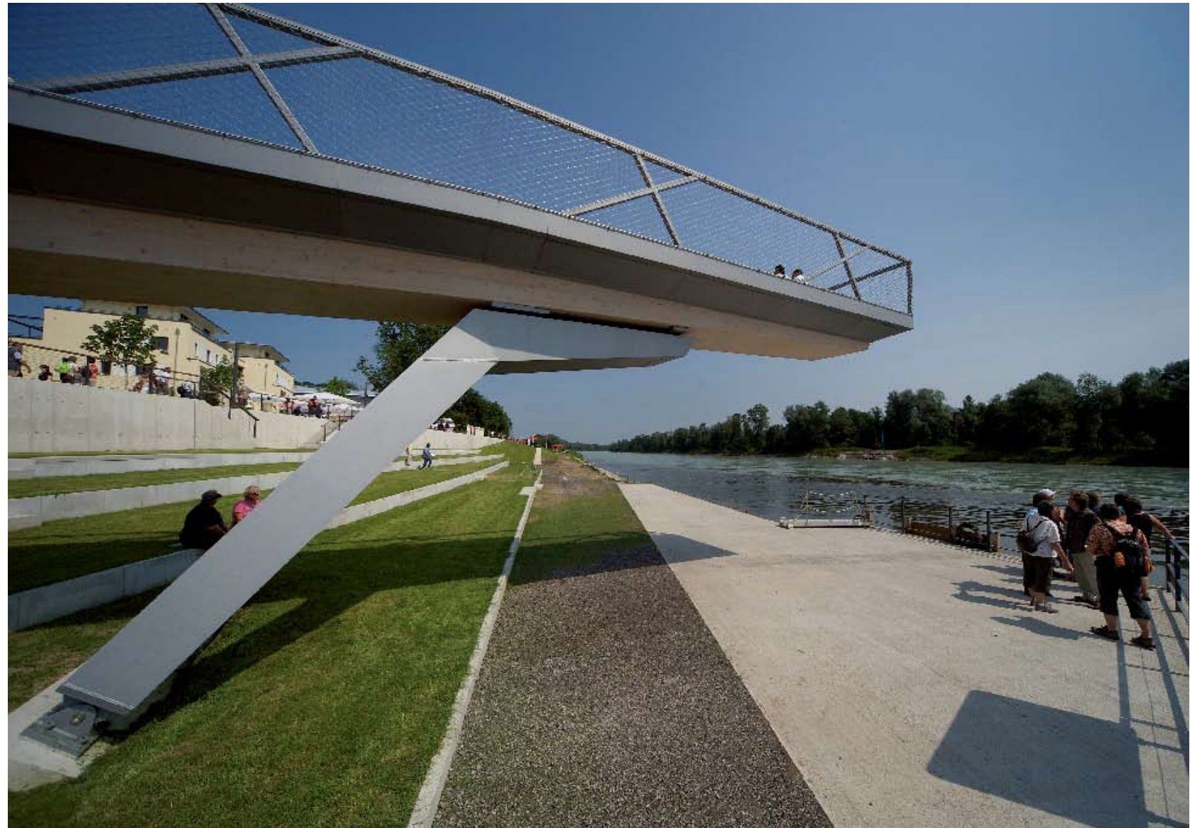
Left: Top view of the Mangfall Bridge Upper right: Terraced lawn elements at the lookout point Lower right: Entry area to the kayaking route at the Hammerbach creek
