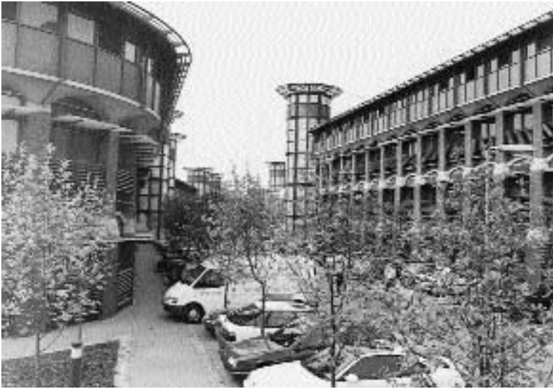
Figure 4.14 Canalside development, Nottingham: The Inland Revenue Building by Michael Hopkins and Partners.
