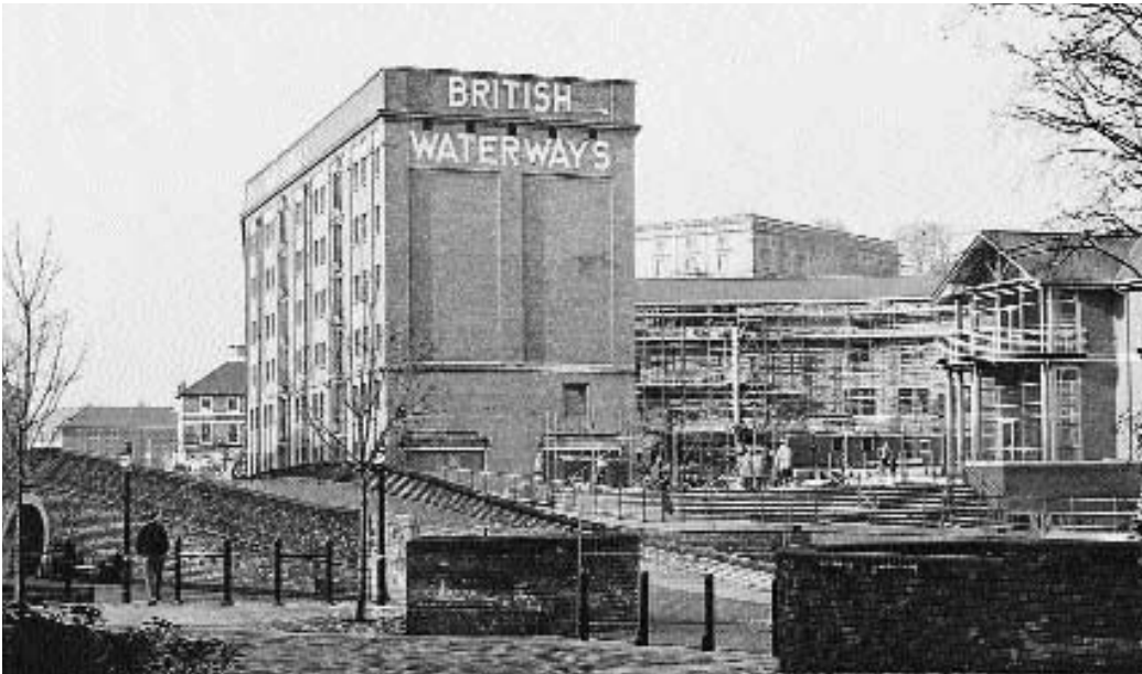
Figure 4.16 Canalside development, Nottingham: refurbished warehouse.
