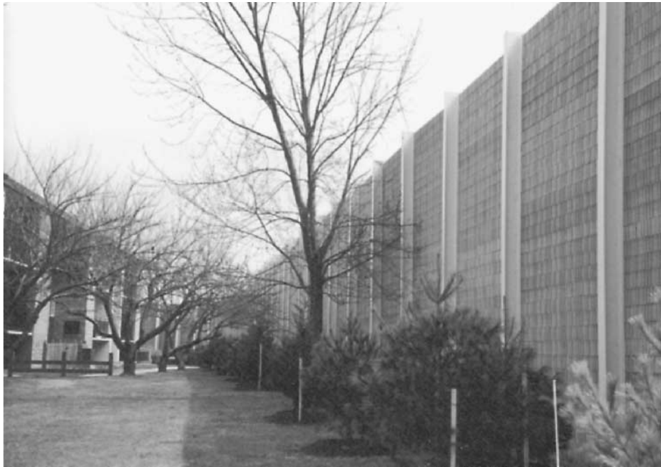
Figure 3.8 Photograph of sound walls.
