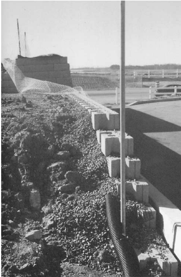
Figure 3.16 Photograph of interlocking walls.
