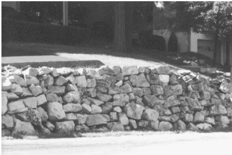
Figure 3.20 Photograph of dry laid stone wall.
