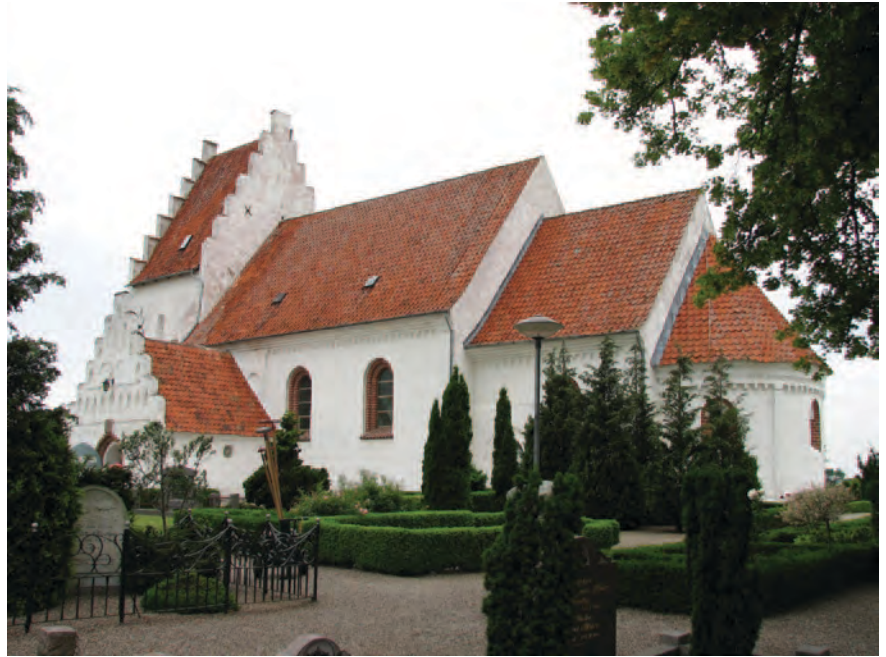
Figure 1. Brarup Church. A typical Danish parish church. The nave and chancel are Romanesque. The tower and porch are Gothic additions. ©National Museum, 2008.
