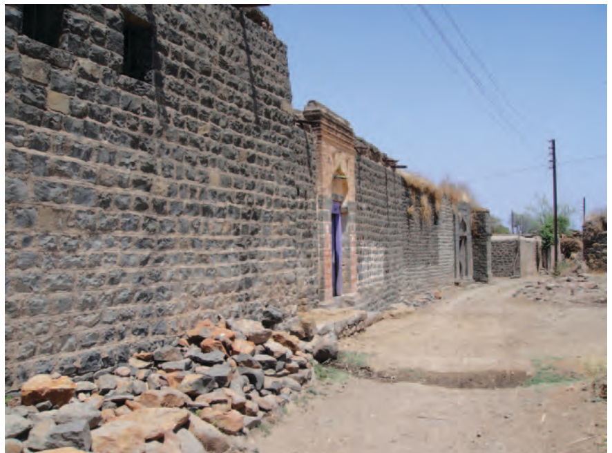
Figure 1. Traditional houses in the region are characterized by massive stone masonry walls, punctuated by large gateways.
