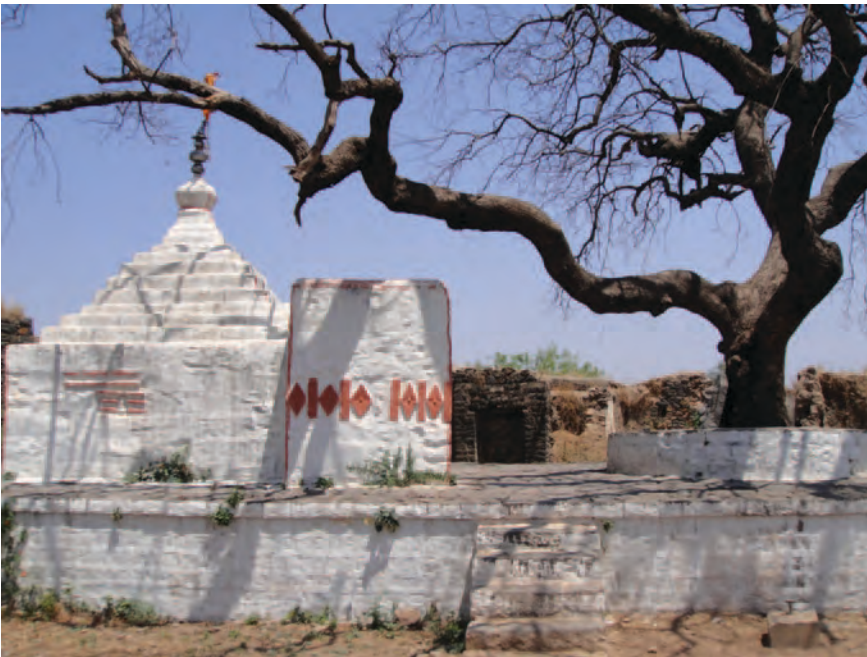
Figure 3. Stone temples with a typical pyramidal roof made of corbelled masonry are typically found at the entrance of every traditional village.
