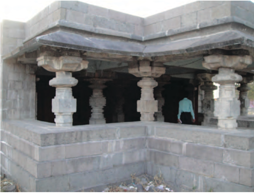
Figure 2. Very sophisticated dry stone masonry can be found in some historic temples in the region such as this one near Killari town.
