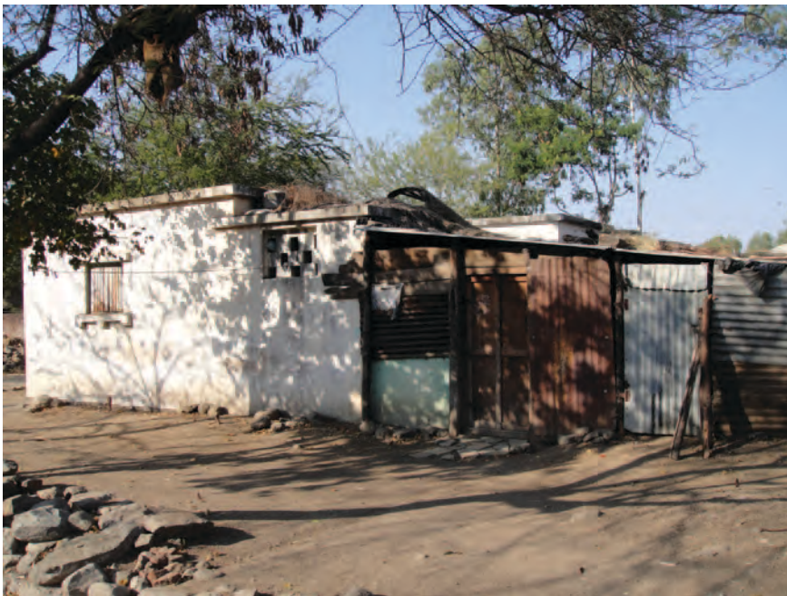
Figure 10. In many cases, people have used cheap corrugated tin sheets to make additions to their reconstructed houses.
