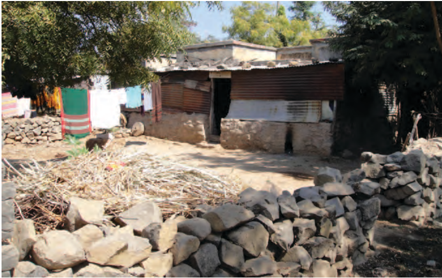
Figure 9. Stone in random rubble masonry is only used for making boundary walls.
