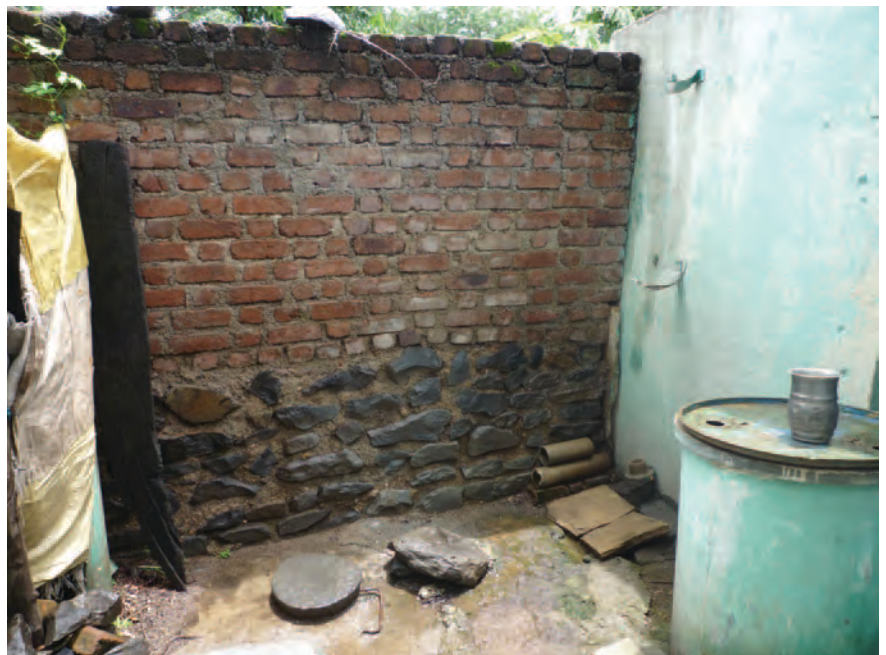
Figure 12. Many additions made for outdoor kitchens are in poor brick masonry, covered by tin sheets that can easily blow away during heavy winds.
