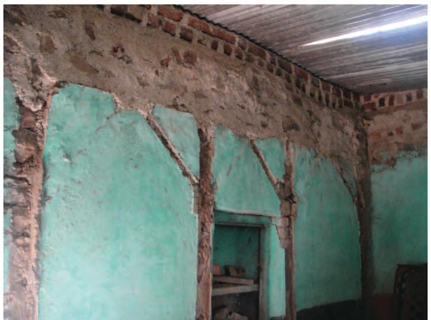
Figure 15. The iron angles used for retrofitting traditional houses have been removed to increase the ceiling height. Moreover, the traditional roof, made of wooden beams and rafters, is being replaced by tin sheets.
