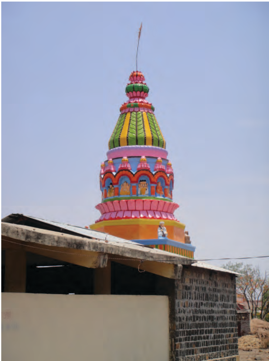
Figure 16. Traditional stone temples that were considerably safer against earthquakes have gradually been replaced with reinforced concrete structures of poor quality, built with new architectural techniques from the surrounding region.
