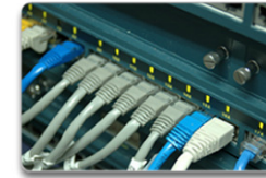
Cables must be connected correctly.
