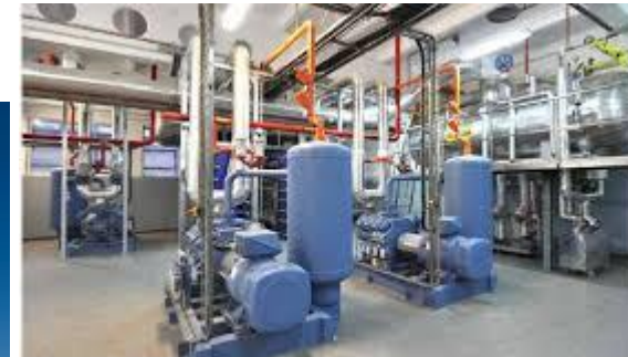
With the aid of GEA Grasso V1100 piston compressors and an automatic GEA Grasso control system, a Polish dairy co-operative increased its refrigeration capacity by 25% with the same power consumption
