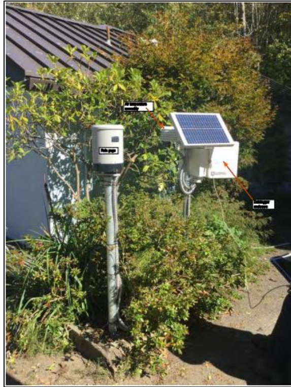
Figure 7.5: Typical rain gauge installation including an enclosed datalogger and temperature sensor assembly (Smith et al., 2017)
