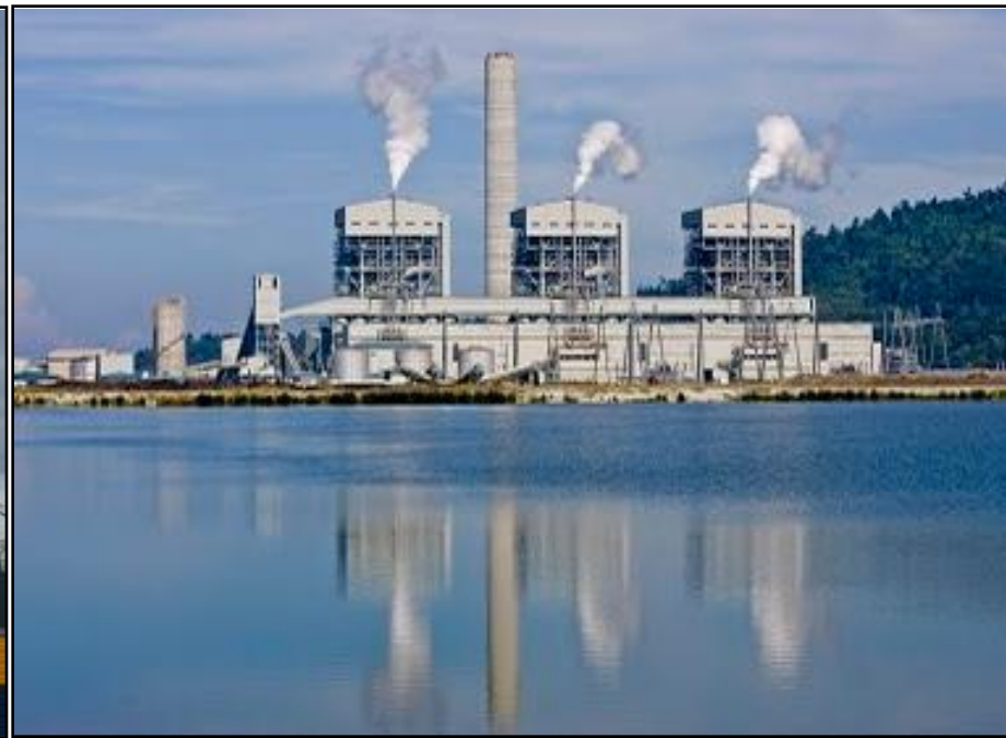
Power plant site in Manjung Perak
