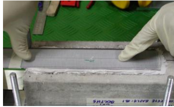
Fig. 3(a): Pressing the CFRP plate onto bond surface to remove excessive epoxy mixture.
