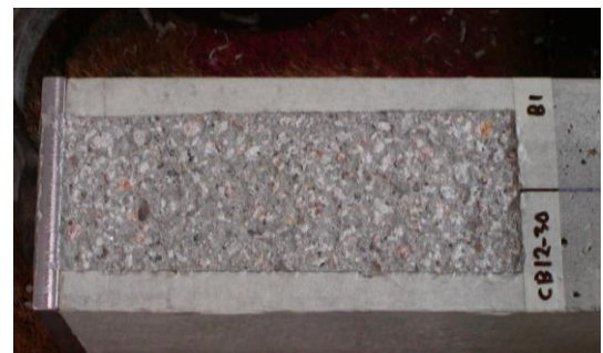
Figure 1: The roughened surface of concrete prism
