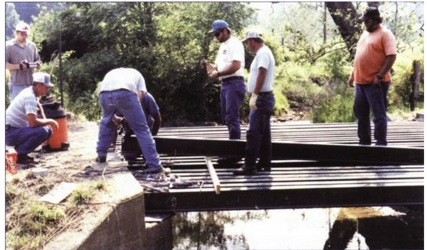
Steel flange beams were replaced by pultruded FRP beams, reinforced with carbon fibres in the flanges to increase stiffness to over 6 million psi, in this bridge upgrade in Blacksburg, Virginia.
