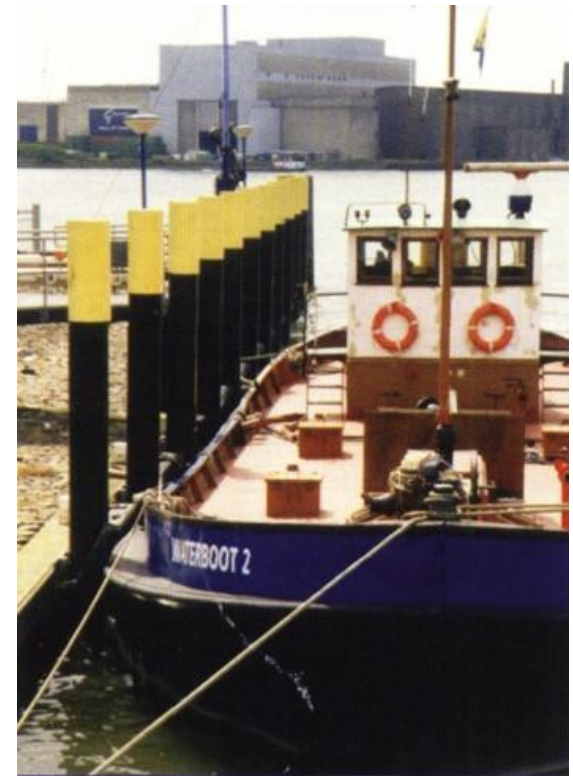
Composite piling being used for a dock installation in Rotterdam. (Picture courtesy of Seaward International/PC Jansen Marine Agencies.)
