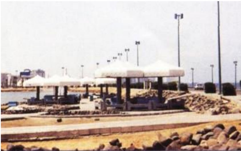
FRP light poles and GRP shading and seating at Jeddah Corniche, Saudi Arabia.
