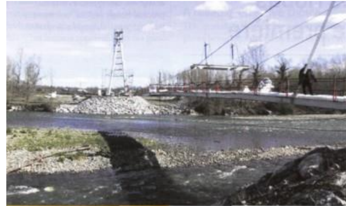
The Laroin footbridge is the very first in France to use carbon-fibre composites.
