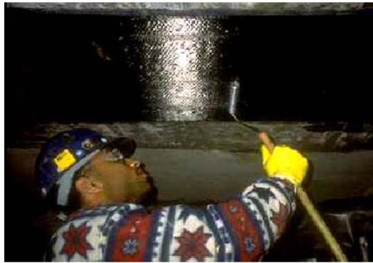
Fig. 2.2: FRP laminate system used for strengthening RC beam [7]
