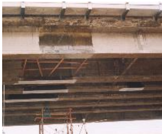
Fig. 2.3: Muar Bridge Beams strengthened with CFRP Sheet [2]
