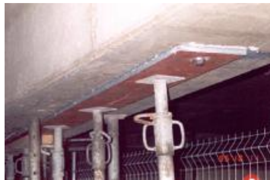
Fig. 2.1: Steel plate member used for strengthening RC beam [4]
